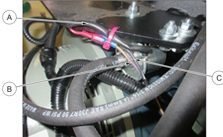
Figure 3 - Fuel Pump Wires
